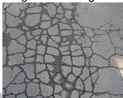
Alligator Cracking
